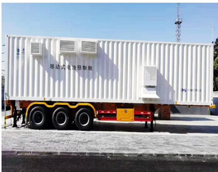
Mobile box energy storage system in Yanqing substation, Beijing
