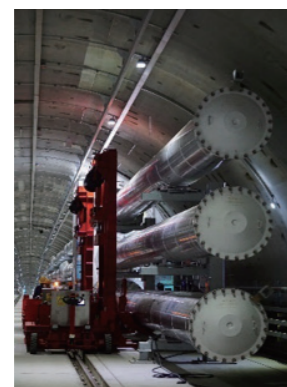
GIL tunnel installation vehicle
