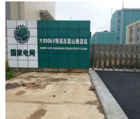
Shaoshan converter station
