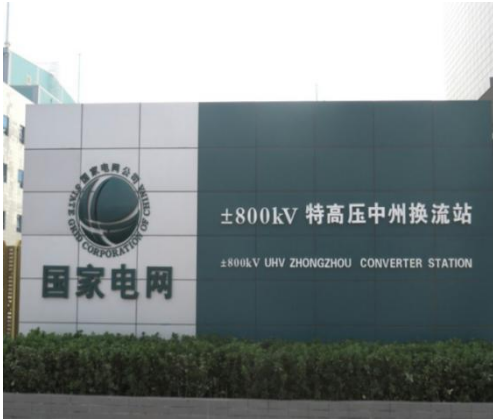
Zhongzhou converter station
