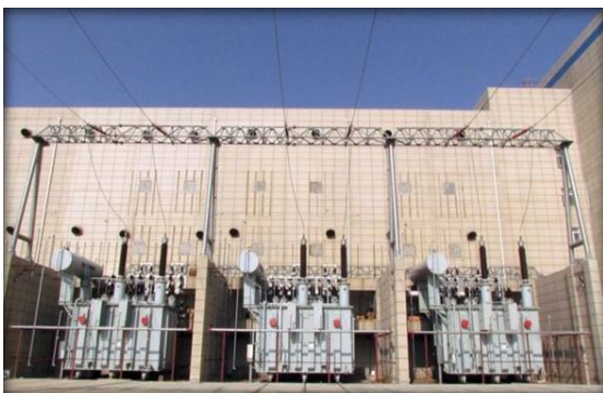
Short-circuit test transformer
