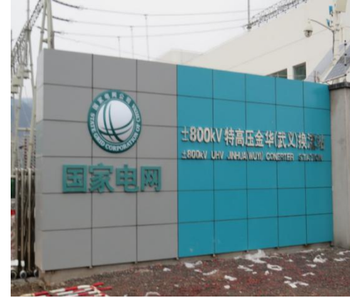
Jinhua converter station
